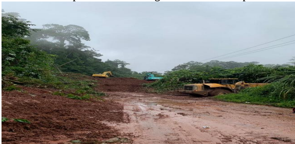
Public Works and Transport sector: Repaired road and pre-assessment
